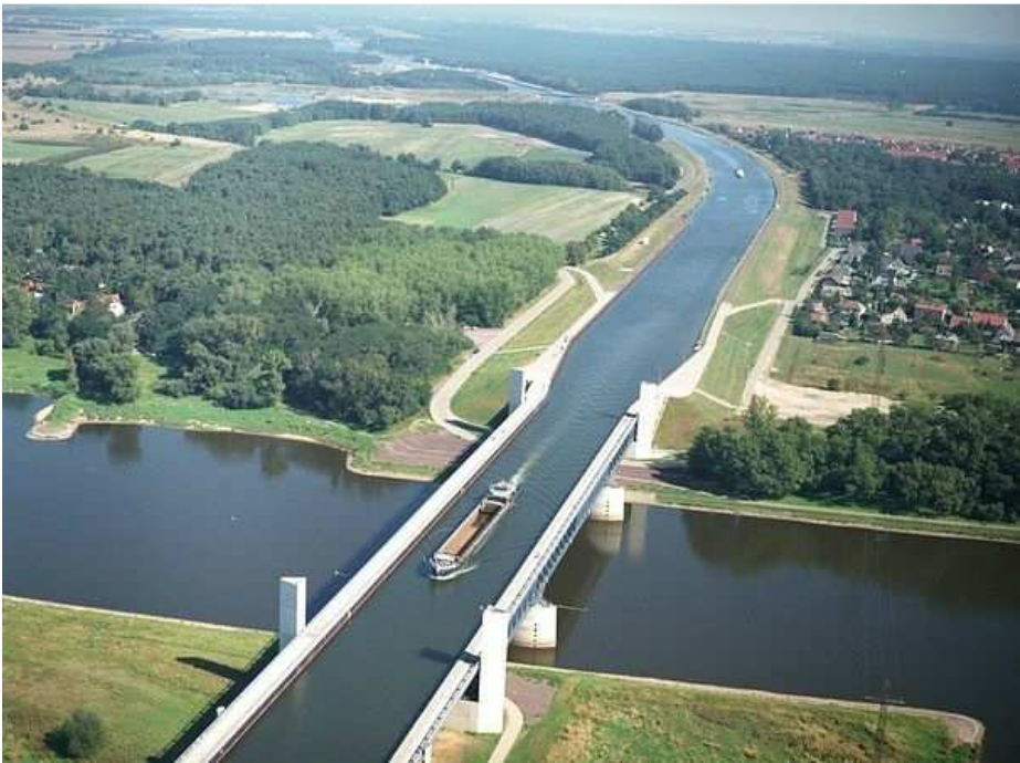
The river above the river: Magdeburg Water Bridge, Germany.
