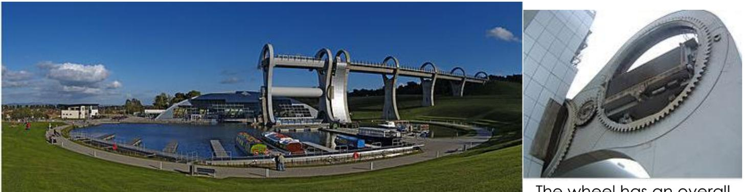
The wheel has an overall diameter of 35 meters (115 ft) and consists of two opposing arms extending 15 meters beyond the central axle and taking the shape of a Celtic-inspired, double-headed axe. Two sets of these axe-shaped arms are connected to a 3.8-metre (12 ft) diameter central axle of length 28 meters (92 ft). Two diametrically opposed water-filled caissons, each with a capacity of 250,000 liters (55,000 imp gal; 66,000 US gal), are fitted between the ends of the arms.
